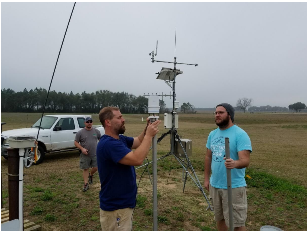
Below: John and Matt (Vellidis' crew) installing Atmos weather station.
