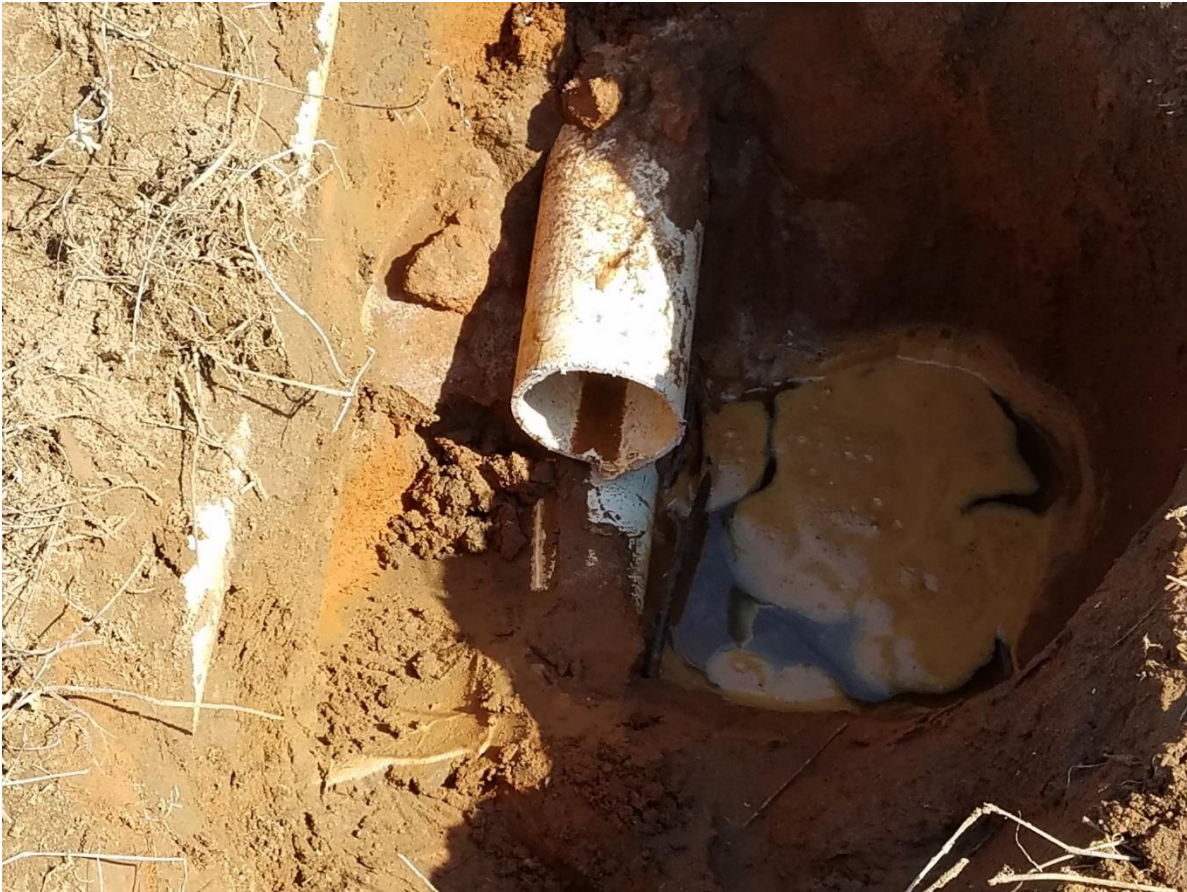
Above: Having to repair busted water line.
