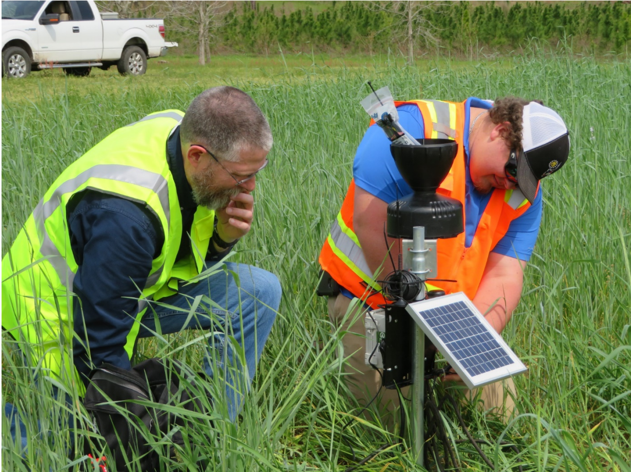
Above: Dan and Hunter installing Valley soil moisture sensor in Rye in our “Newton” linear-move field.
